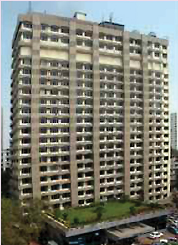
Jaslok Hospital - Mumbai
